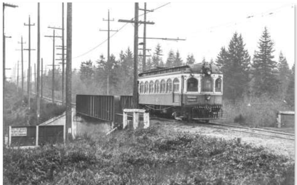
Figure 220 ~ Pershing Bridge, looking southwest toward the undeveloped Westminster Triangle neighborhood. (SHM-1412)
