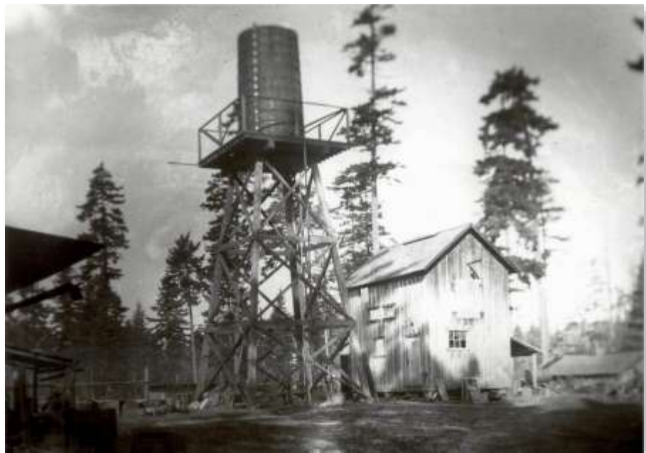
Photo 209 ~ 1910s. Schneider's water tower and pump house stood in Richmond Highlands at 180th and Aurora for many years. The water tower was later enclosed for a shop. This site became the location of the Highland Ice Arena in 1962. Photo donated by Richard Schneider. (SHM-2016-G)
