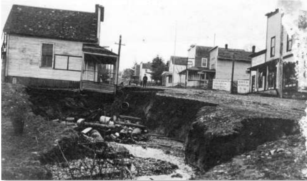
Photo 198 ~ 1916. A remarkable snowstorm followed by flooding in some areas brought a substantial washout to Market Street in Richmond Beach. The immense runoff from a culverted stream could not be contained by the pipes. The small café at the corner of Market and Charles St. was a victim of the event.
