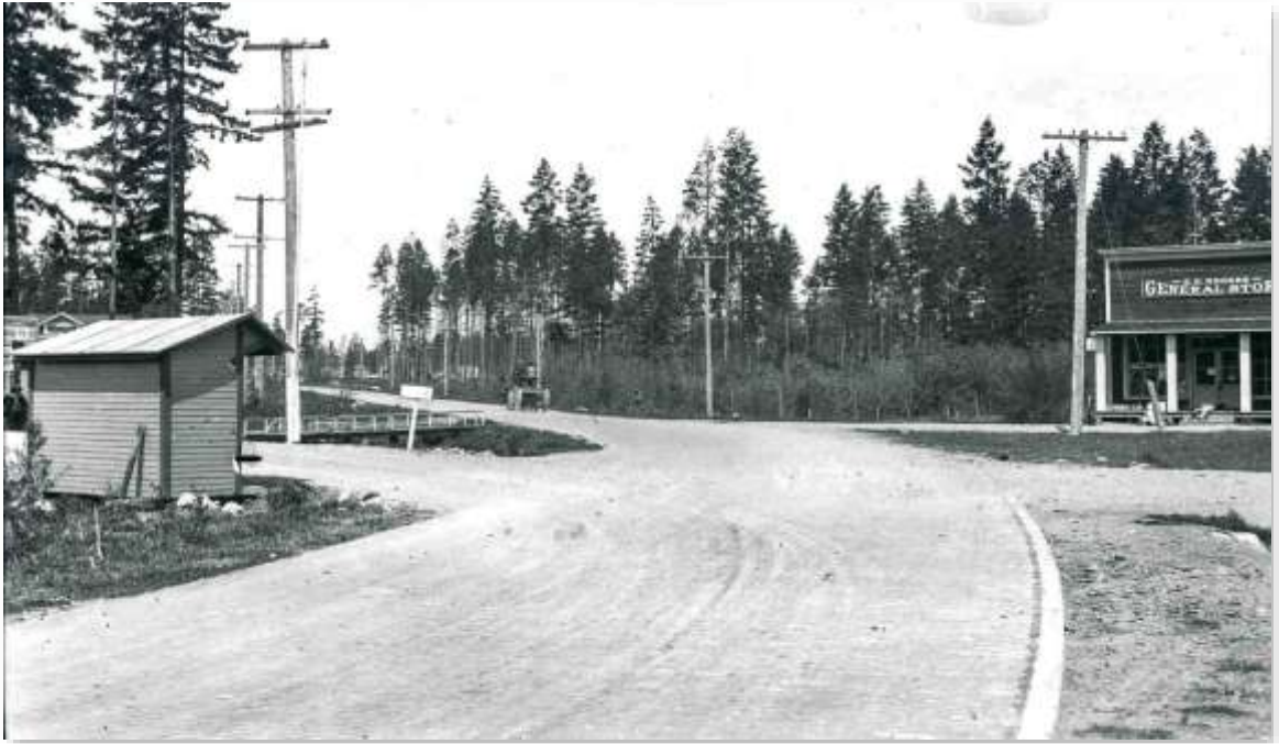
Photo 16 ~ ca. 1914. Looking north on the North Trunk Road where it becomes Firland's Way at N. 185 th Street, which crosses left to right at center. The new Biles house on Firland's Way is barely visible in the background over the top of the bus stop shelter at the far left. Courtesy King County Archives.
