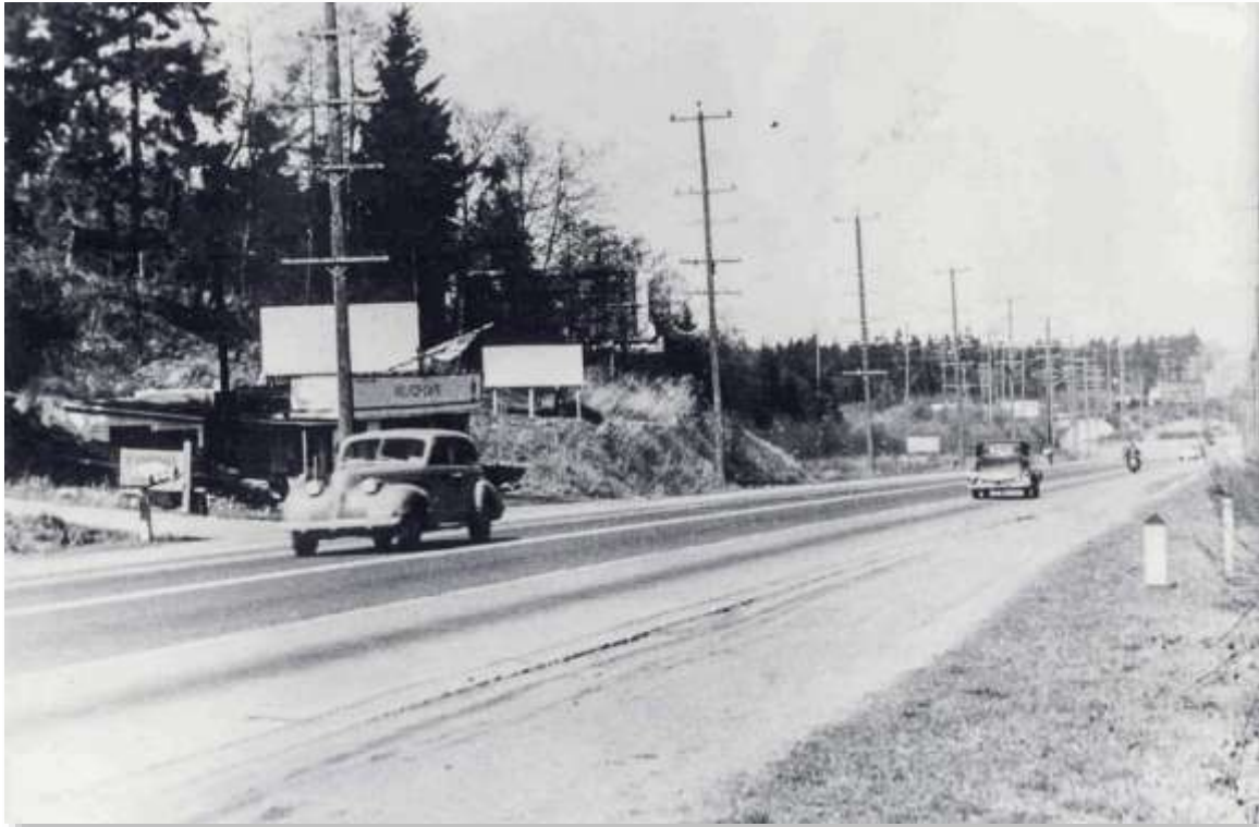
Photo 221 ~ 1932. The Hilltop Inn and the dirt road entrance to the Skyline Auto Court on Aurora Avenue. (SHM-257-B)
