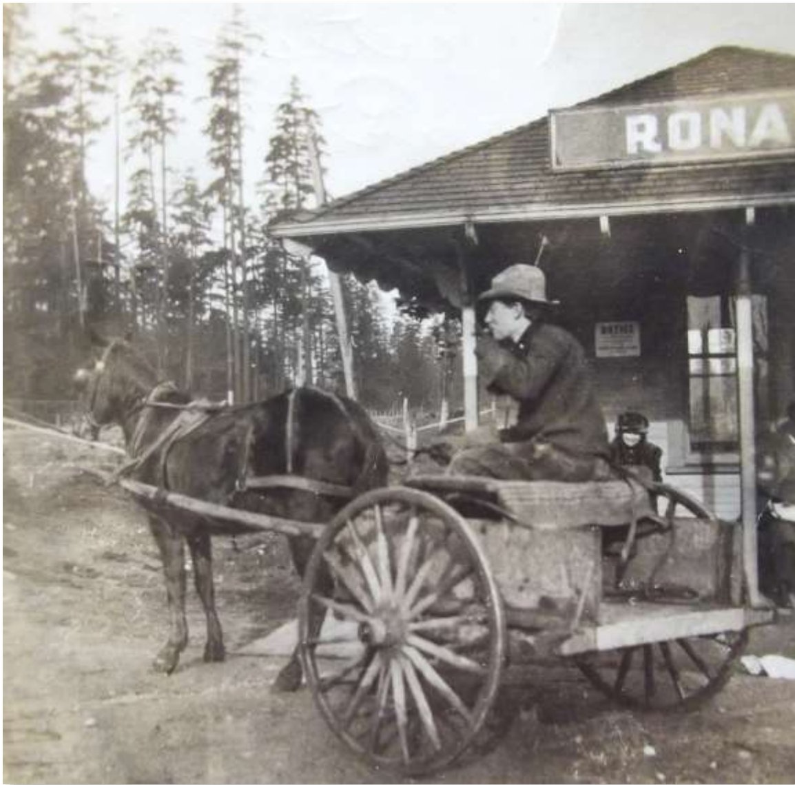
Photo 86 ~ ca. 1920. At the Ronald Station, Morton Clark Sr. sits in his wagon after delivering a relative. The trolley right-of-way has been regraded, and the station lowered to track level. At the far left is 175 th St. marked with a fence along its south edge. Donated by Morton Clark Jr., Morton Clark Collection.
