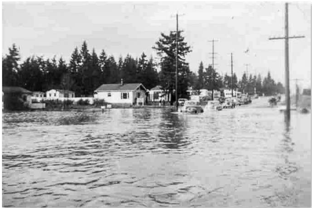
Photo 57 ~ ca. 1953. Flooding on Aurora was an almost annual event after land was cleared around 1945 at what would become the Sears and Roebuck site near 155 th and Aurora on Westminster Way. The scene is from near the intersection of Aurora and 160 th . Donated by Bud Wilkinson. (SHM-3183)
