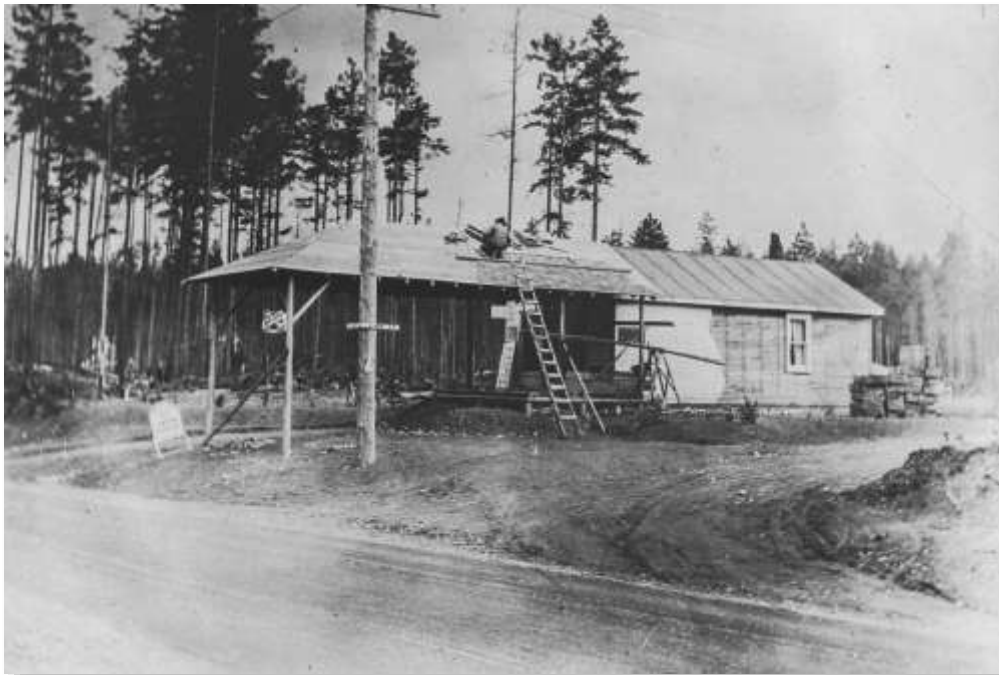
Photo 69 ~ 1928. Edward Yenn's Monte Vista Grocery and Gas was strategically located on 15 th Ave NE at about 165 th . The street sign says N. 164 th , a street that does not exist today, or ever in this location. It was the closest store to the new Monte Vista development which was highly advertised. (SHM-345)
